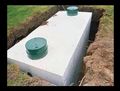
Septic tank size is determined by design flow – number of bedrooms for residential systems Minimum size septic tank = 1000 gal (Required for 4 bedroom and smaller homes) Add 250 gal for each additional bedroom over four
