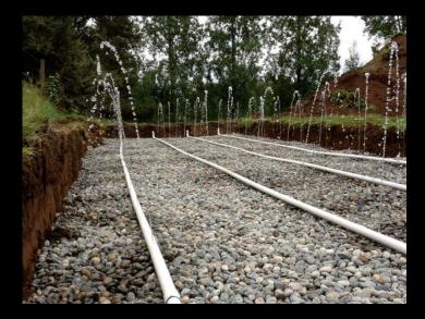
Leach field size is determined by wastewater volume to be infiltrated and the permeability of the receiving soil. Low permeability soils require larger area to absorb a given volume of wastewater.
